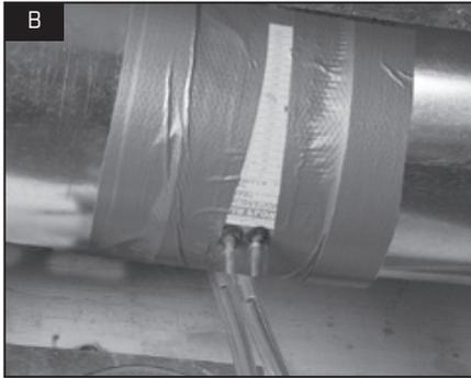
**1** For this flow measuring station, cut the duct and place the flow measuring station between each section of duct. Make sure that the flow measuring station's air direction arrow points in the direction of the airflow. Secure the flow measuring station with duct tape.
