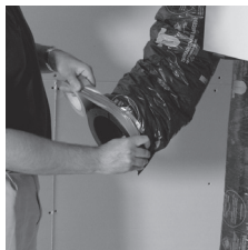
Finish by taping the vapor barrier to the collar to insure proper seal.
