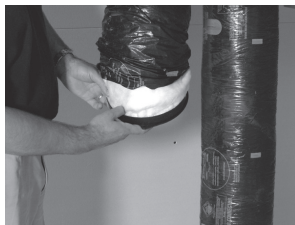
Insert insulation inside the double collar.
