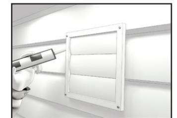
**1** Using the duct connection of the outside hood, outline the intake & exhaust holes to be cut. The holes should be slightly larger than the duct connection to allow for the thickness of the insulated flexible duct. Cut a hole for both the intake and exhaust hoods.
