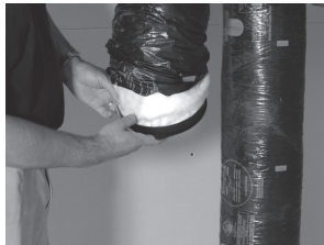
Insert insulation inside the double collar.
