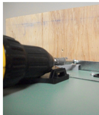
figure 6.4 Proceed to secure HRV/ERV to bracket with the two #8 x 3/8" screws.
