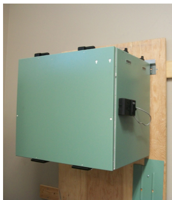
figure 6.2 Hang HRV/ERV to wall mounting bracket.
