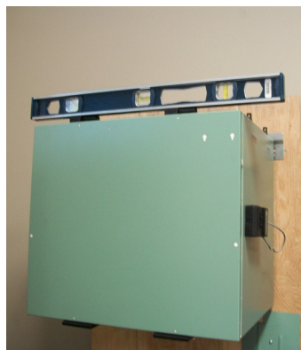
figure 6.3 When completing the procedure make sure that the HRV/ERV is leveled.
