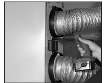
Figure 7.5 Fix and secure with two screws supplied.
