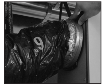
figure 7.4 Slide collar on the unit.
