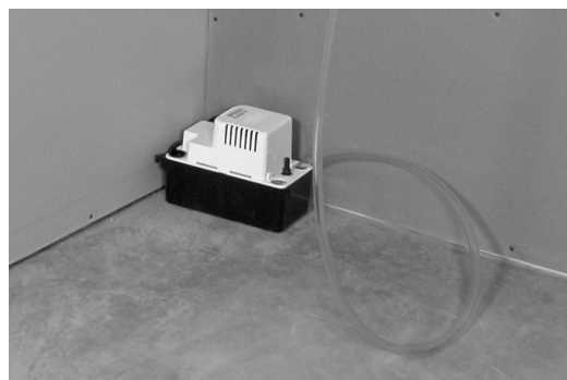
figure 9.2 Use a condensate pump if you don't have access to a drain.
